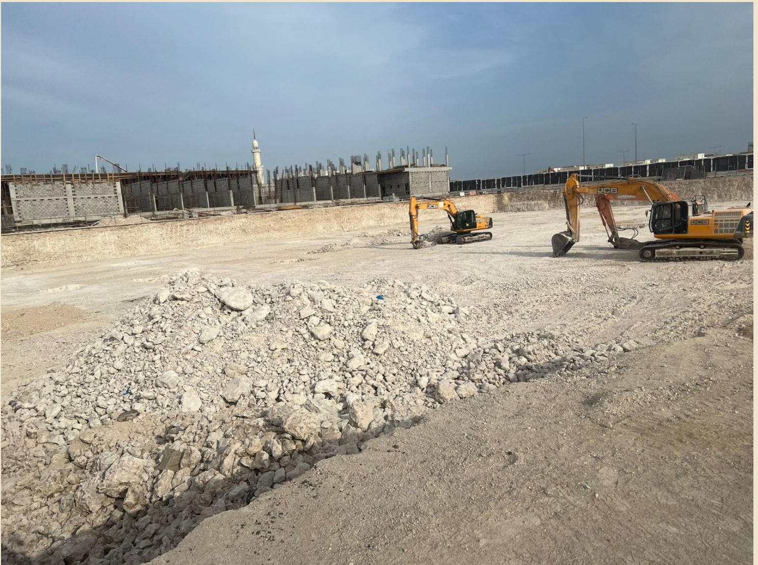
Excavation and leveling works for the Al Wukair project, 2025
