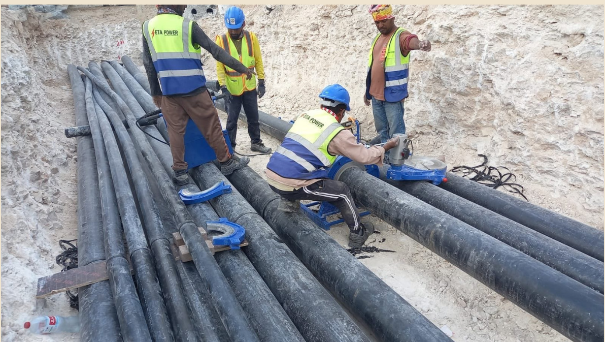
Excavation and extension works in Al Kharaitiyat, Al Darwish Engineering, 2025.
