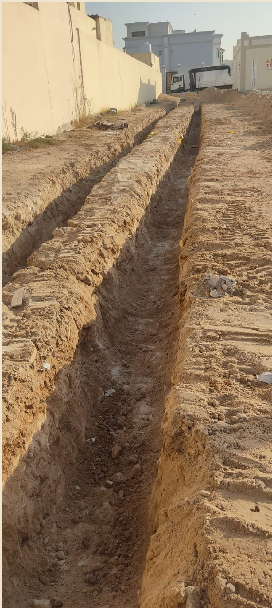
Excavation, leveling, and extension works in the Unaizah, QBC, 2024-2025
